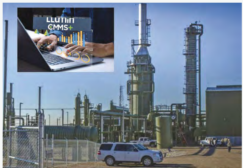
FIGURE 1. Integrating its CMMS and control systems helped Red Cedar Gathering's treatment facility increase its uptime above 99%.
