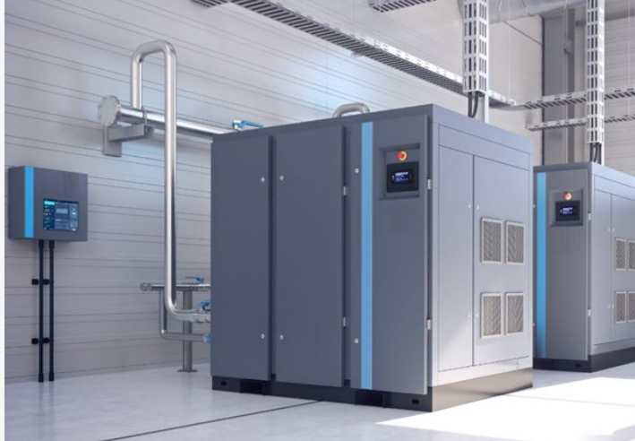
FIGURE 1. Carefully selecting compressor sizing and control method can ensure efficient system operation. Compressor room piping should be sized for minimum pressure loss and should be arranged to ensure good air quality is delivered to downstream components like dryers and filters.
